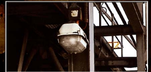
Smooth outer surfaces allow the removal of caked-on product for a full return to the original efficiencies
